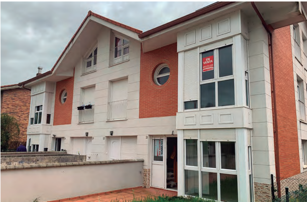
Picture: Façade of an apartment building developed by Sareb in Ampuero (Cantabria).
