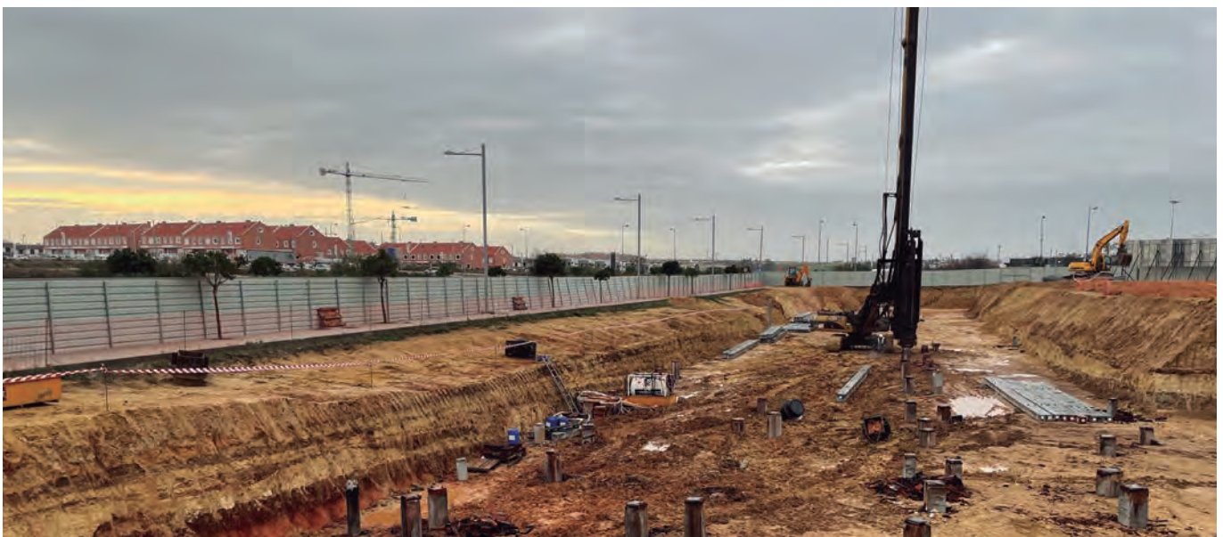
Picture: Construction work at an Arqura Homes development in Seville (Andalusia).
