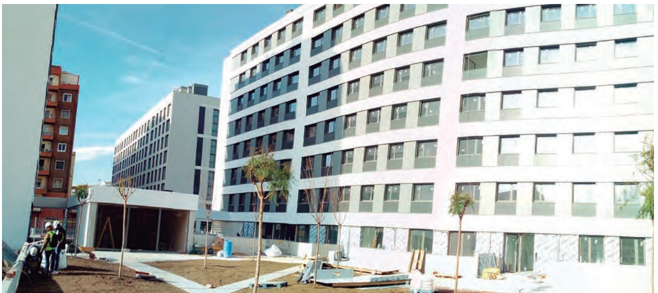
Picture: Apartment building belonging to Arqura Homes in Barcelona (Catalonia).
